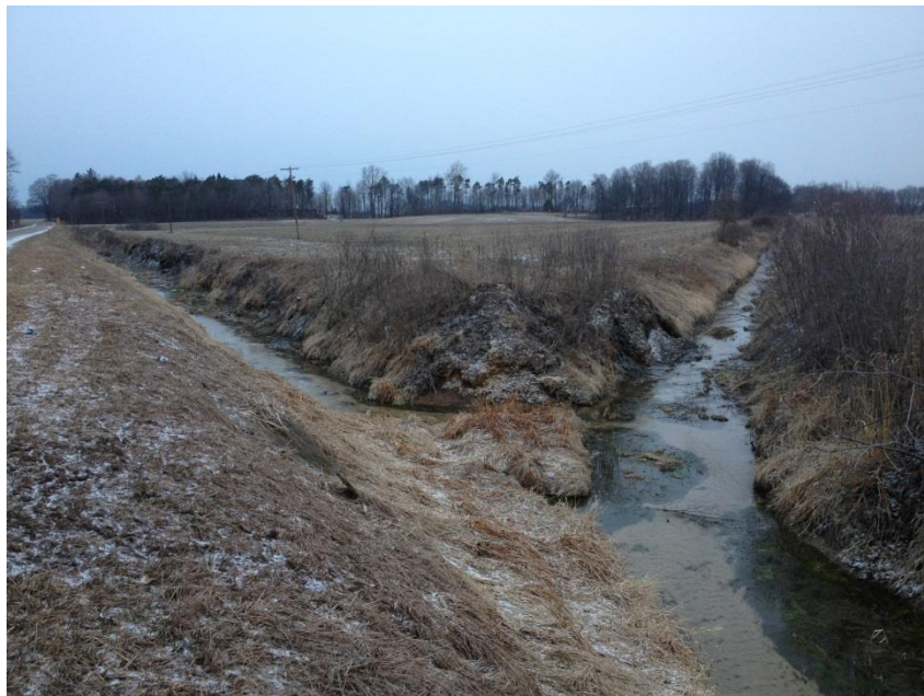
Figure 22: A small tributary along Middle Crossing Rd., just west of the Dowagiac. Sand is present in the channel and during runoff events, it is likely topsoil is being mobilized into the channel as well given the lack of buffer
