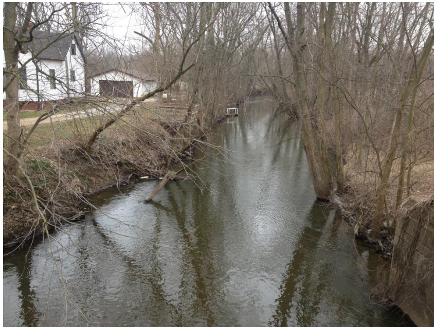
Figure 24: Looking downstream from M-62 at the Dowagiac
