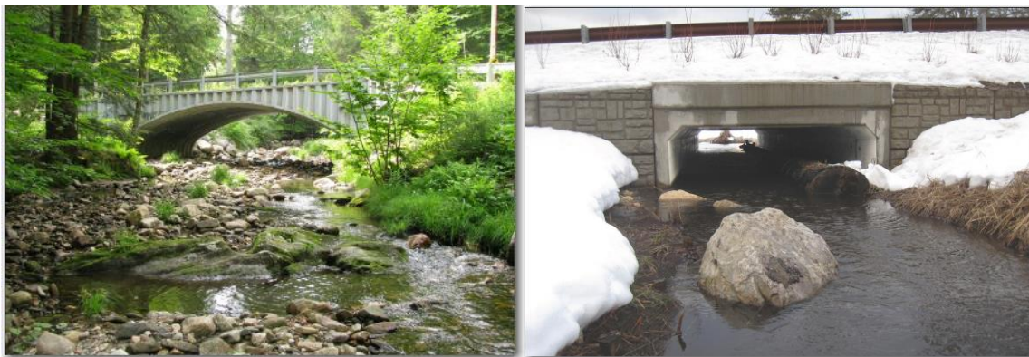
Figure 83. A bottomless arch bridge (left) and a buried concrete box (right) that can be used to replace the existing structure at All Seasons Rd.
