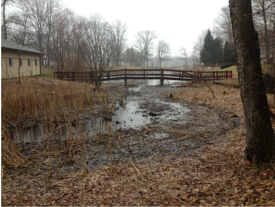
Figure 51. Looking downstream at the Rodgers Pond toward the road
