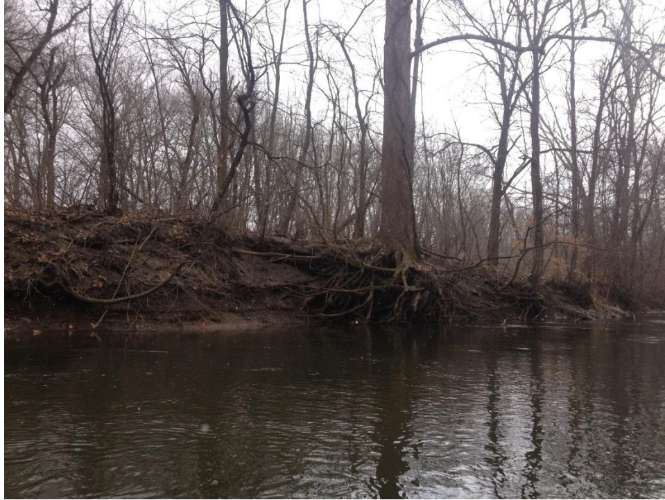
Figure 28. Typical erosion and woody debris along the Dowagiac River banks.
